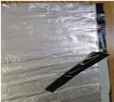
ZIP STRIP OVER ASPHALT EXTNEDED EDGE
